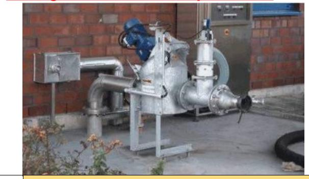
Problem → Blockages and damage to the displacement pumps of the sewage station Solution → VOGELSANG RotaCut<sup>™</sup> 5000 Inline
